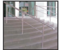
Simple fabrication of handrails for both in and outside.
